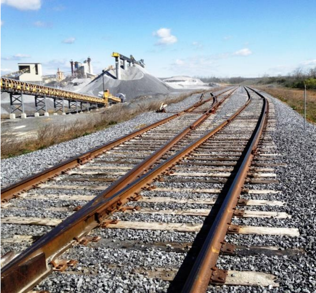
RIA Project: Carmeuse Lime & Stone f Northern Virginia
