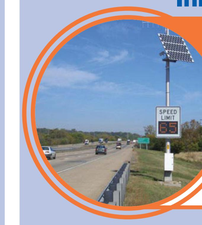
Adjustable speed limit signs that change the speed limit based on the ideal speed to reduce traffic congestion and harmonize the traffic flow.
