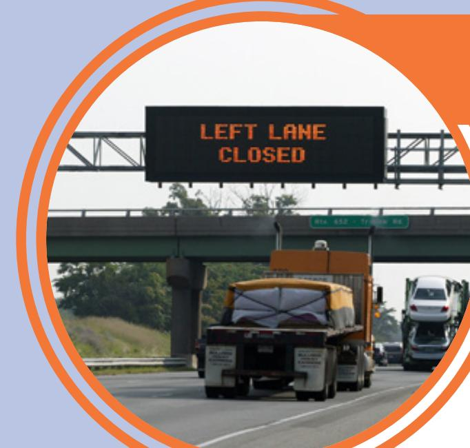
Changeable message signs inform drivers of incident conditions ahead, and can be used to help manage detours.
