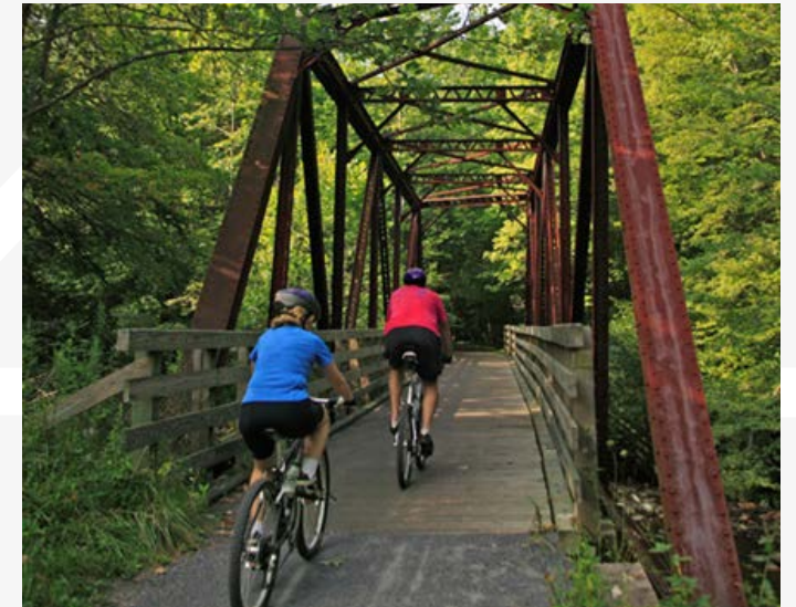
Virginia Creeper Trail, Washington County Source: Toole Design Group
