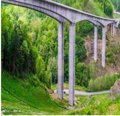
Grassy Creek Bridge (460 Connector)
