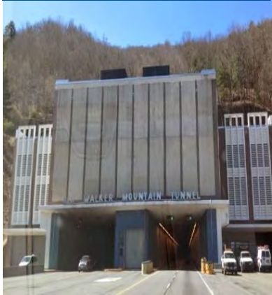
Big Walker Mountain Tunnel
