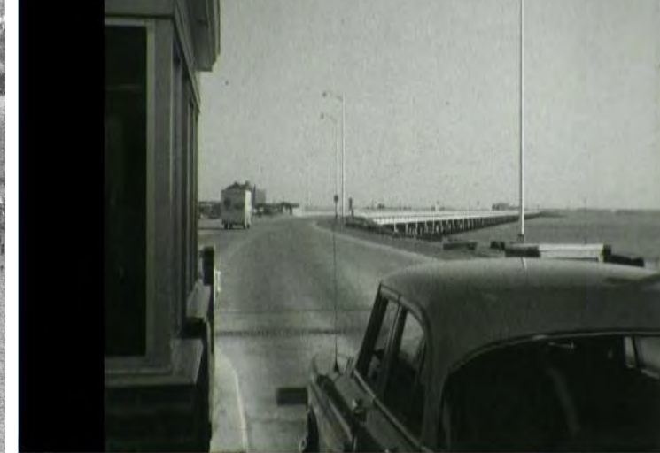
Hampton Roads Bridge-Tunnel
