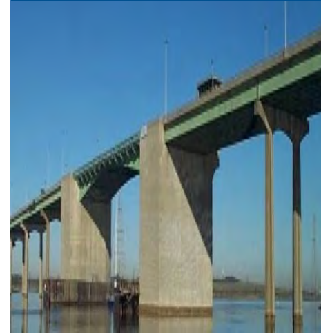
High Rise Bridge
