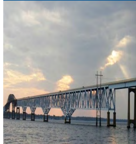
Robert O. Norris Bridge
