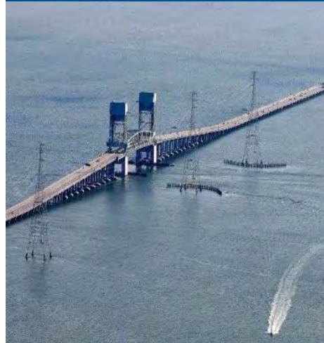
James River Bridge
