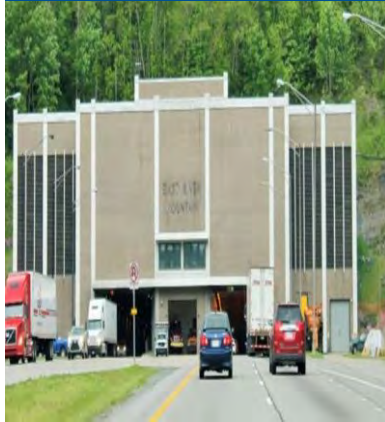
East River Mountain Tunnel
