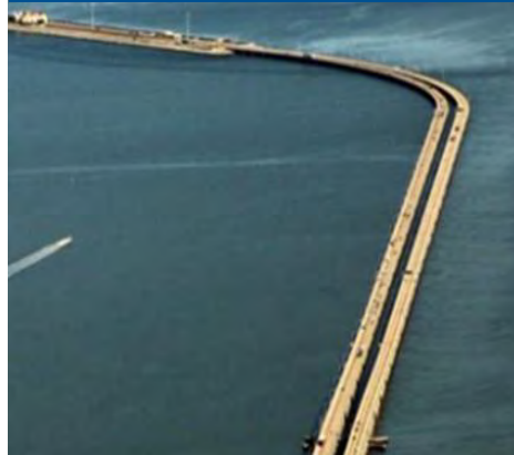
Monitor-Merrimac Memorial Bridge-Tunnel Approach Bridges
