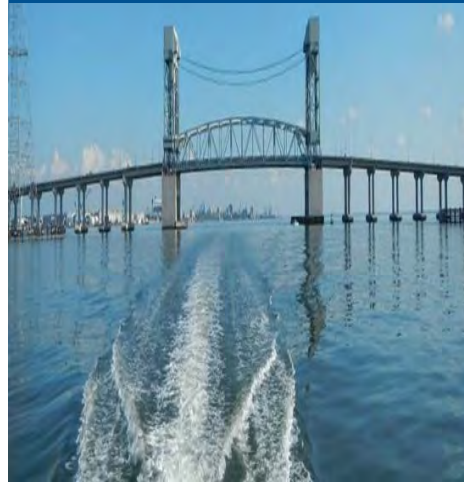
James River Bridge
