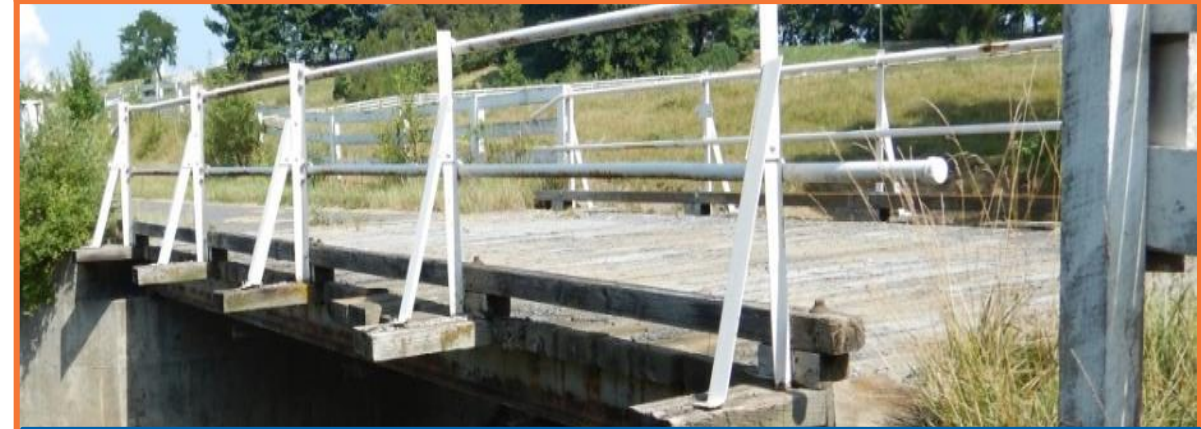
9 Ton Posting – Augusta County Dead End Most School Buses, Fire Trucks, and Ambulances Prohibited
