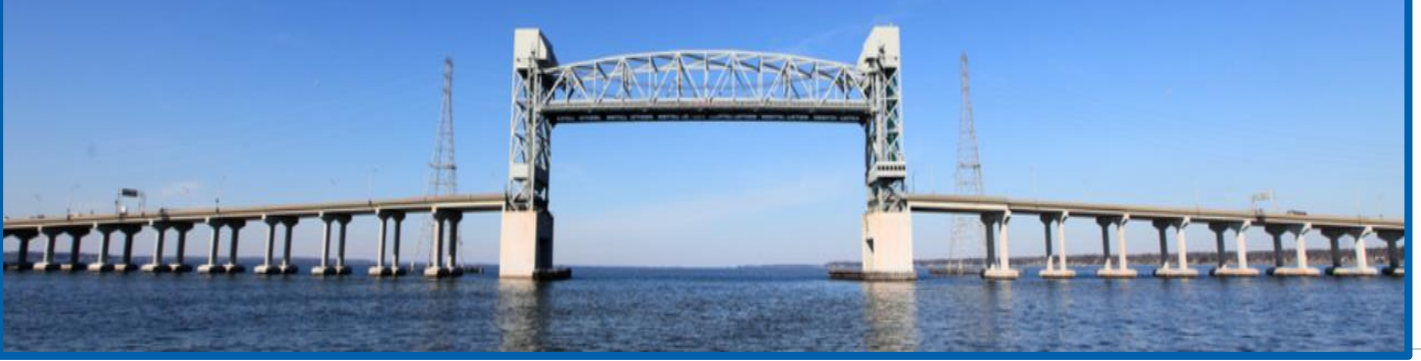
James River Bridge – VDOT's Longest Bridge 4.4 Miles Long
