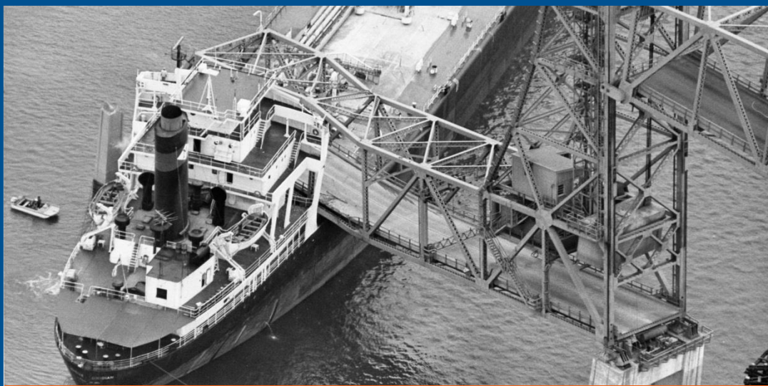
Benjamin Harrison Bridge after 1977 Ship Impact
