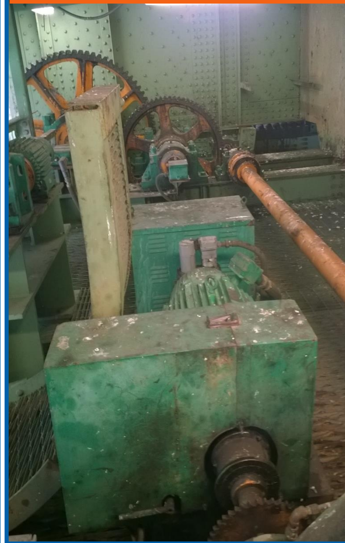
Berkley Bridge Drive Gear
