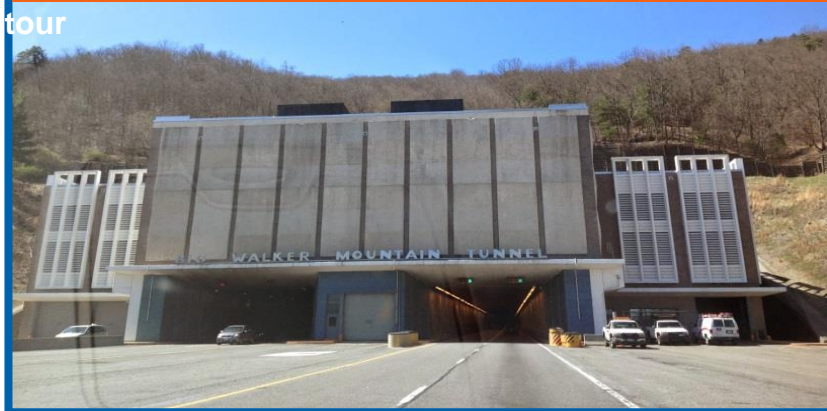
Big Walker Mountain Tunnel Bristol District
