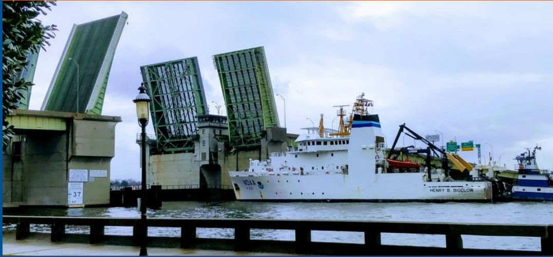
Berkley Bridge – Hampton Roads District
