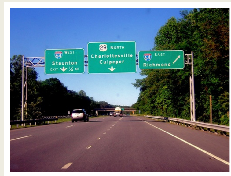
US 29 northbound, south of exit 118
