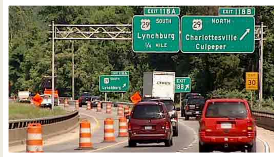
Interstate 64 westbound, exit 118 2011 Bridge Deck Improvements
