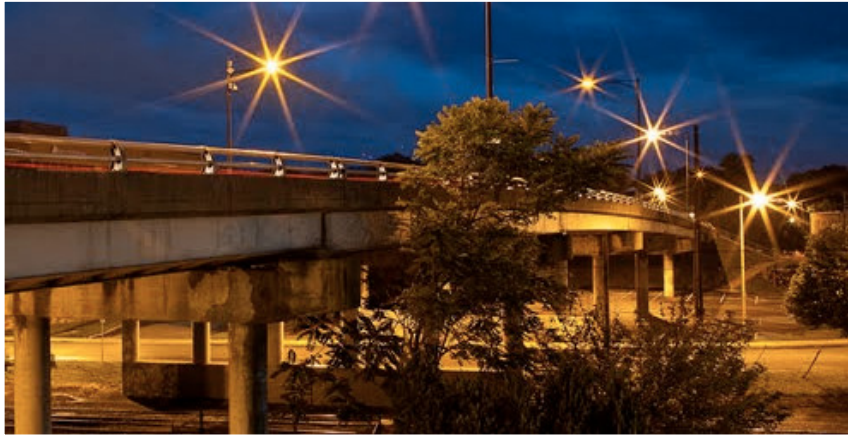
Belmont Bridge - Existing
