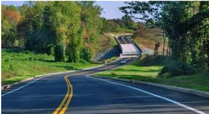
Meadow Creek Parkway – Completed Portion
