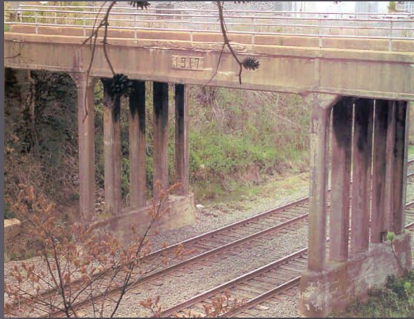
Route 630 Bridge Replacement
