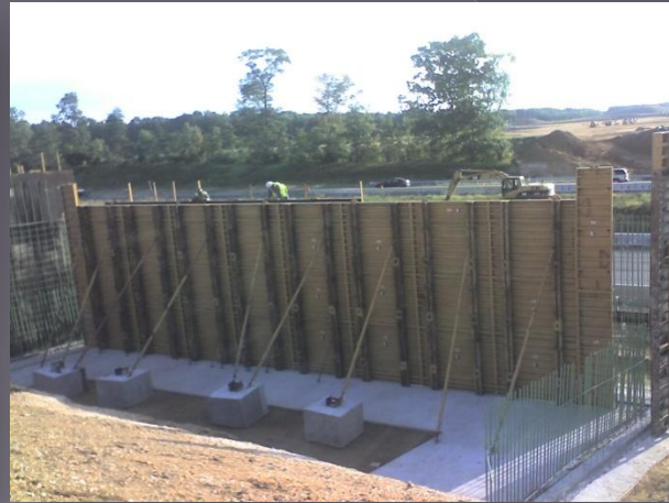
Spotsylvania Parkway Bridge over I-95
