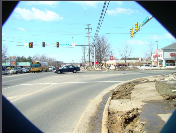
Garrisonville/Onville Rd. Intersection Improvements
