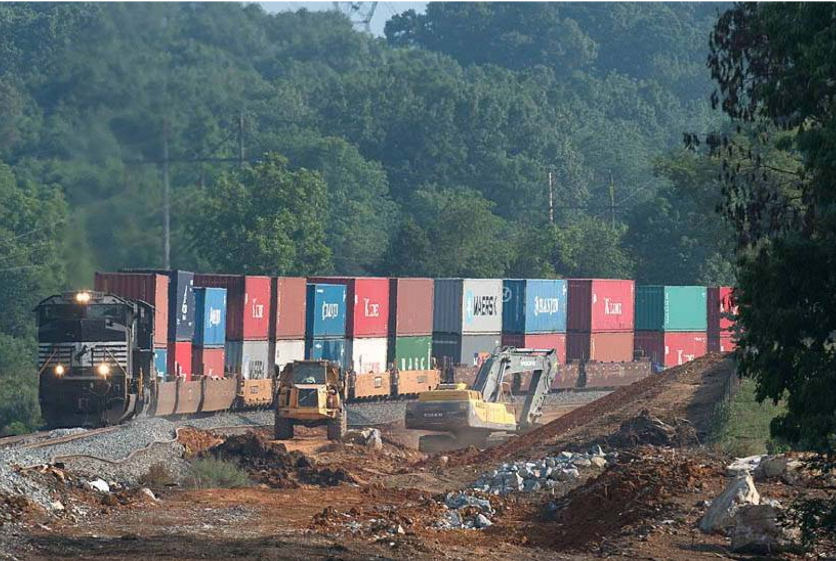
Constructing Roadbed for Second Main Track South of Rockland Road
